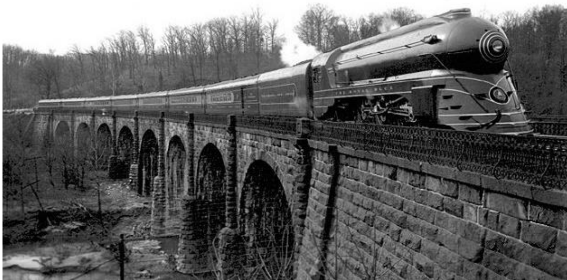
B&O Royal Blue on Thomas Viaduct in 1937 when the viaduct was already over 100 years old. Completed in July of 1835, the curved arch viaduct carries double track mainline CSX traffic to this day.
